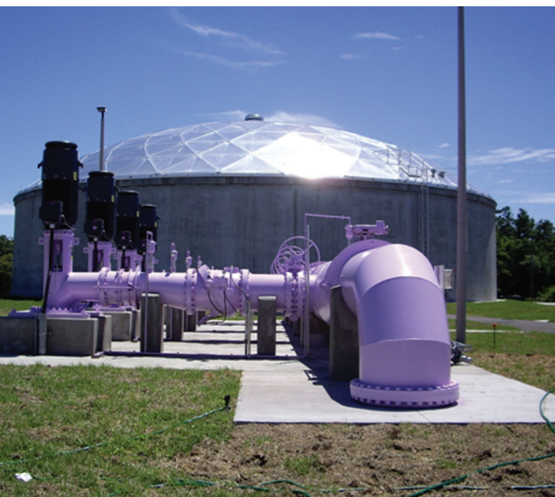
Eastern Orange and Seminole Counties Regional Reuse Project reclaimed water storage tank.
